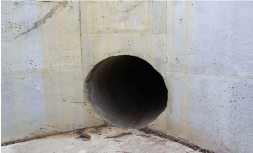
Pipe inlet (western side)
