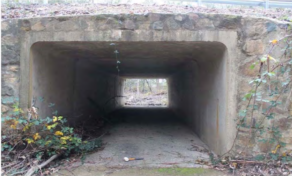
View of culvert from western side
