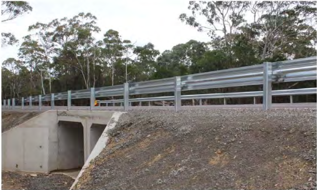
View of culvert from side
