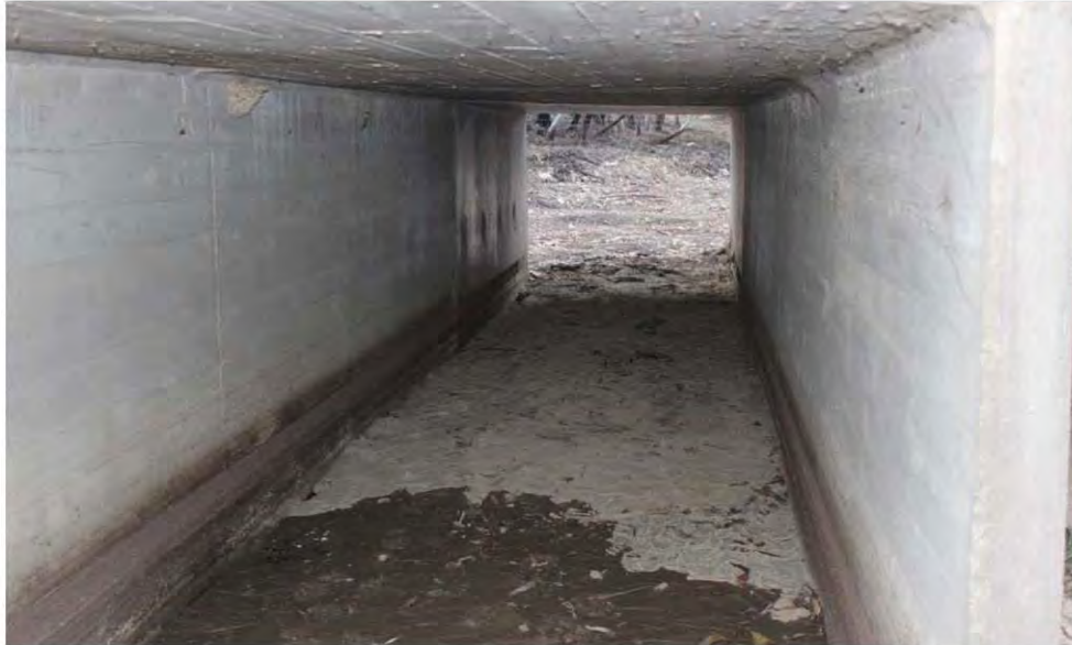
Cell 3 from east
