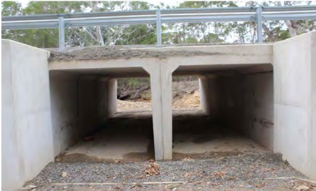
View of culvert from side
