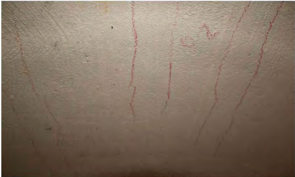
0.2mm transverse cracking in roof
