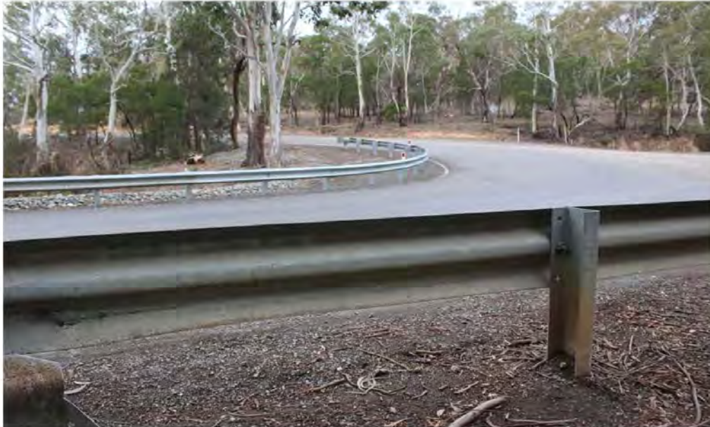
View at road level facing north
