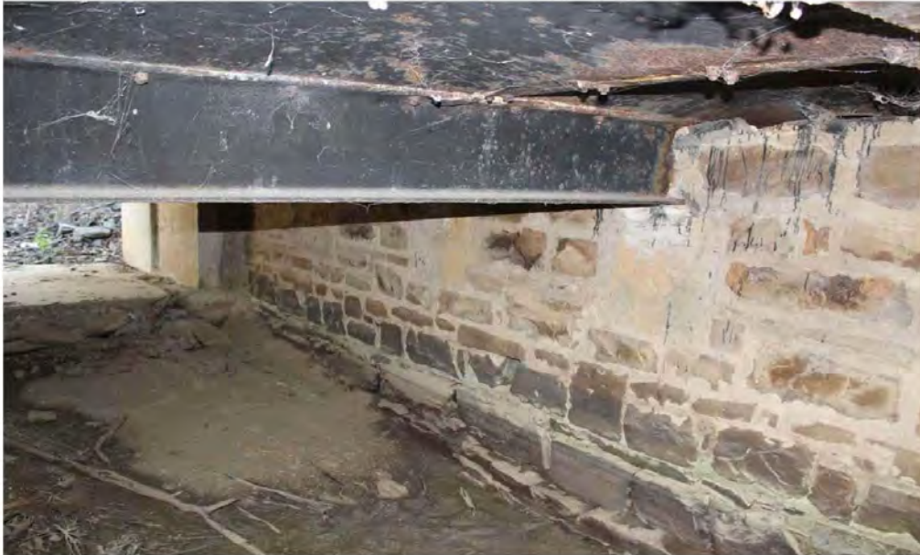
Southern abutment and beam 4
