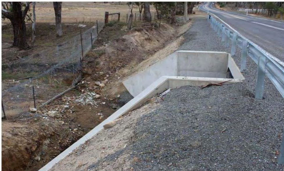
Eastern edge of culvert from top
