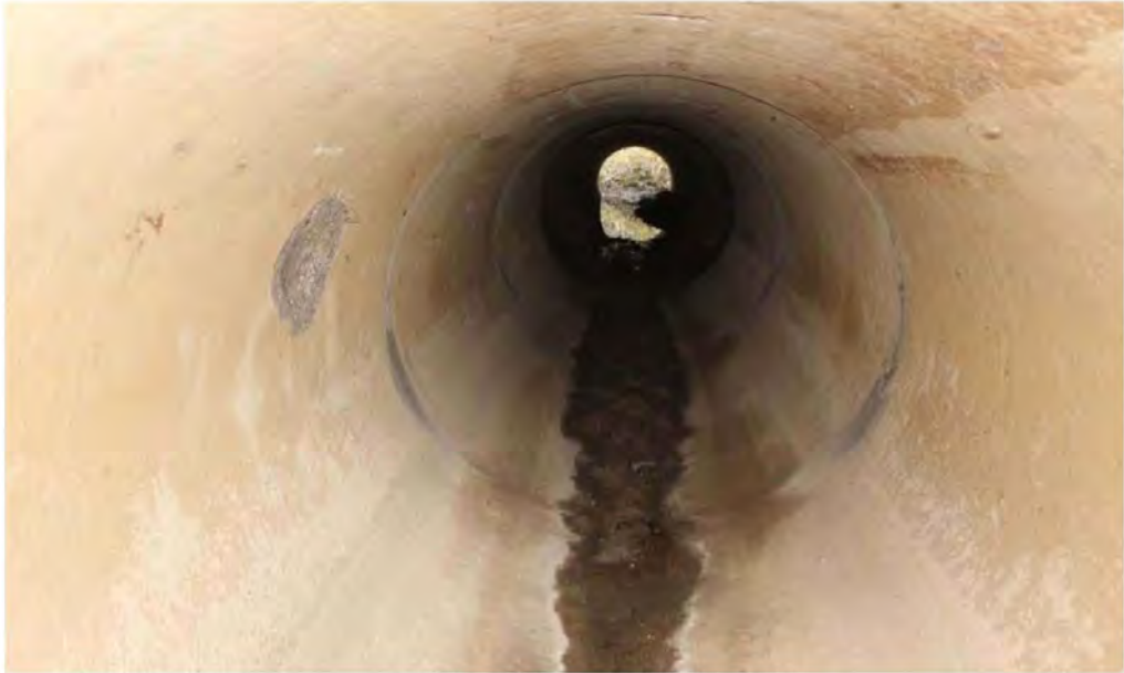
Cell 1 looking south (spall on left)
