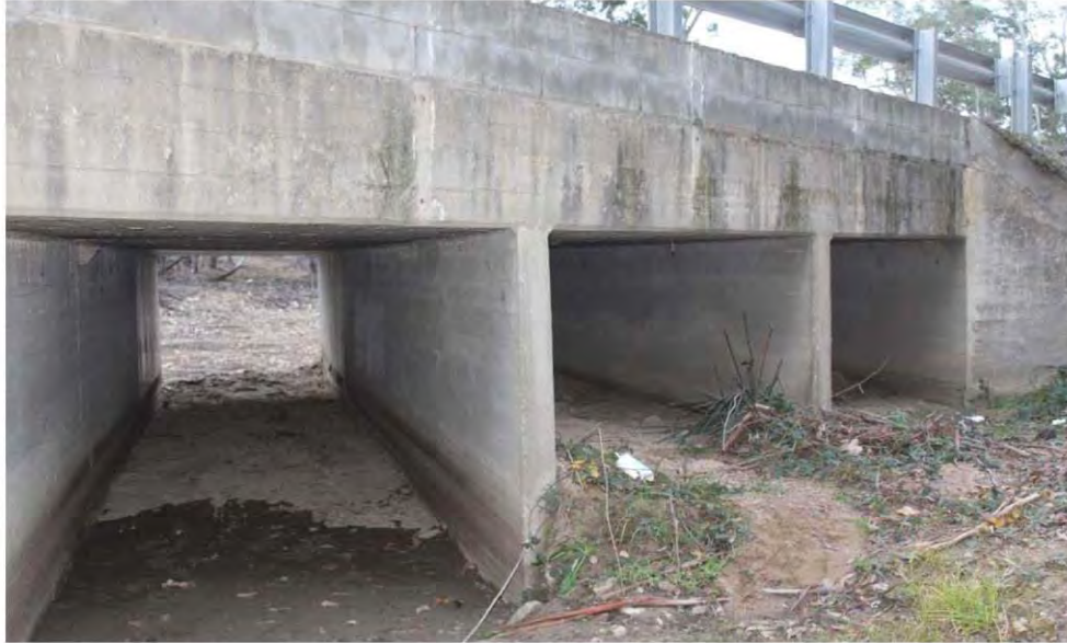
Culverts from eastern side (original)
