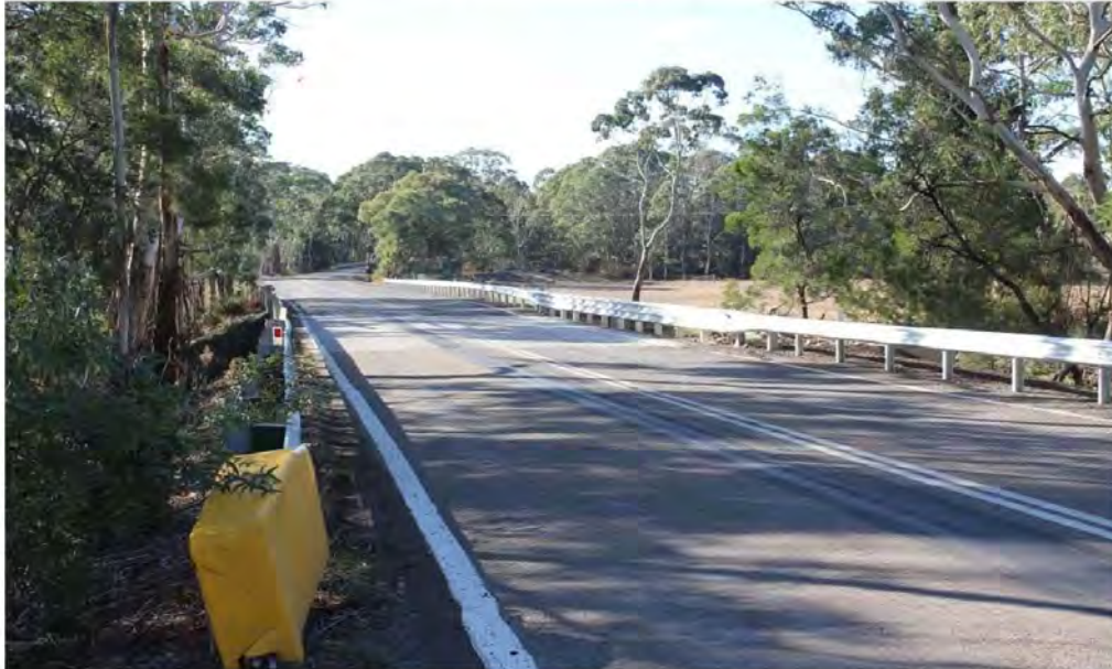
View of bridge from south
