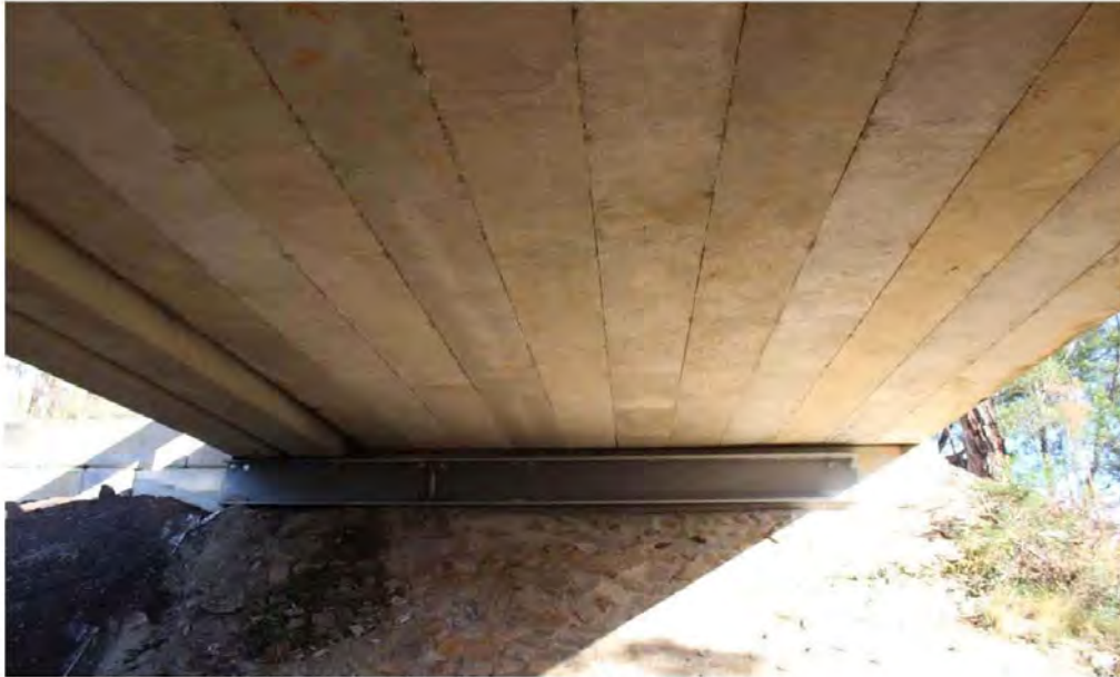
Abutment A and girders
