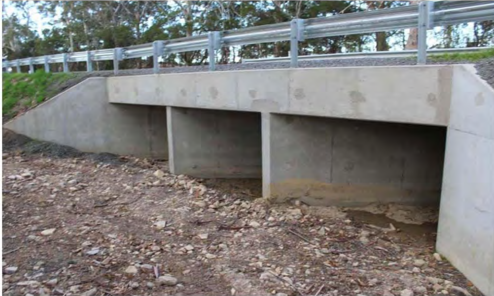
Culverts from western side (recent extension)
