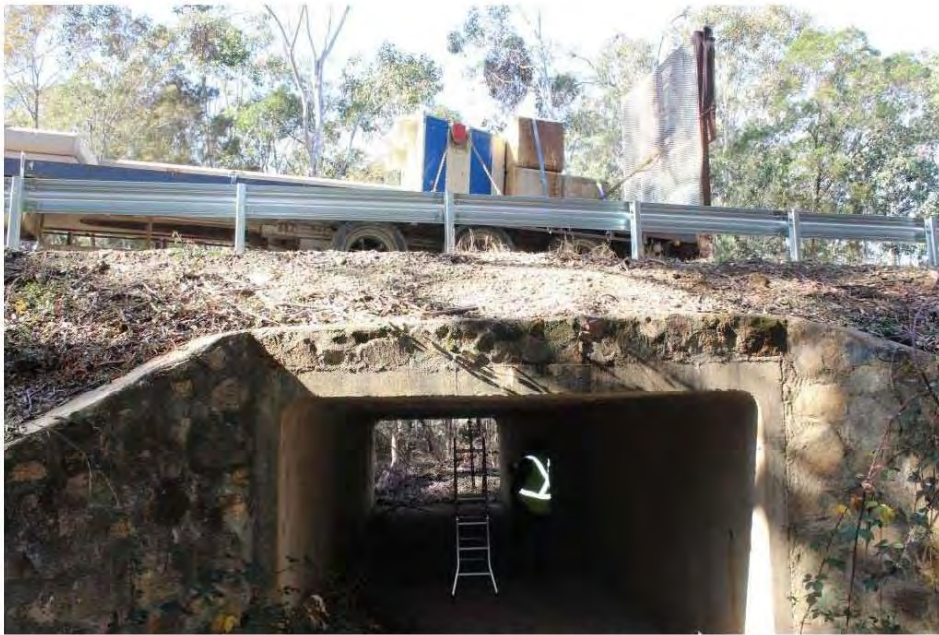
Figure 4.1: Test Setup at Culvert A
