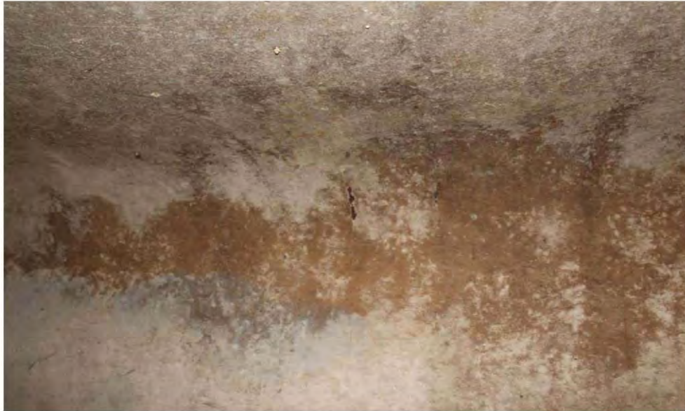
Exposed reinforcement at top corners
