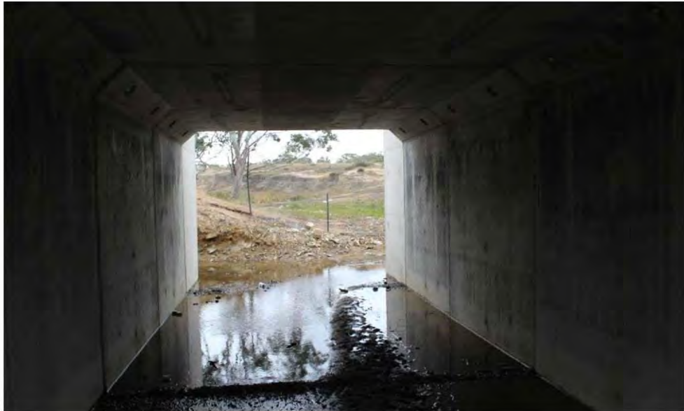
Inside the culvert facing west
