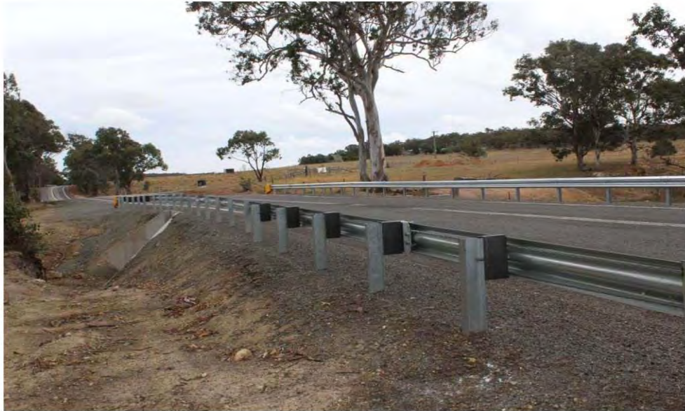
Road over culvert facing south
