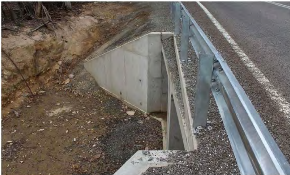
Culvert from road level
