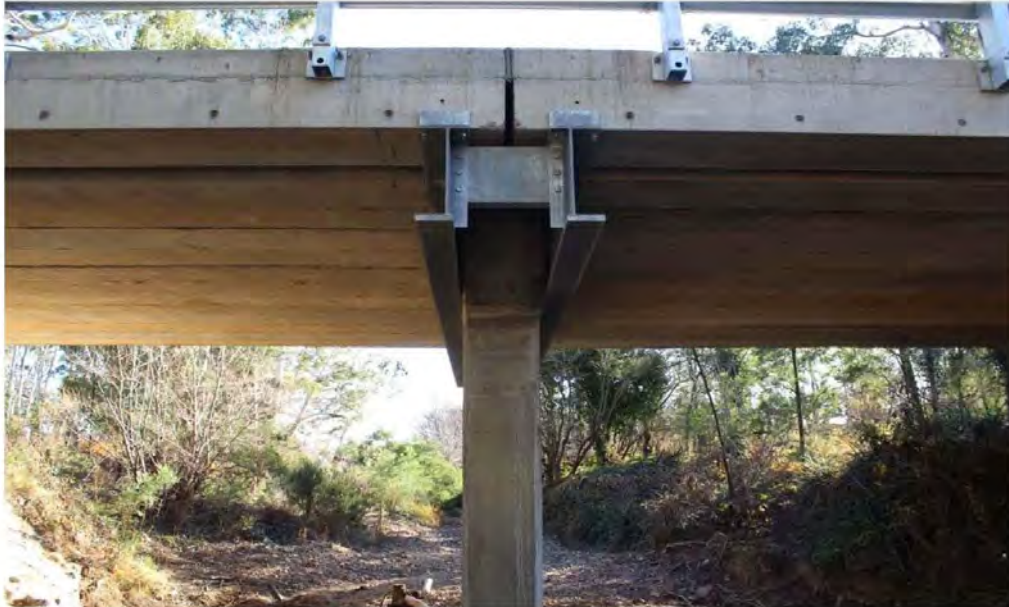
View of pier from east
