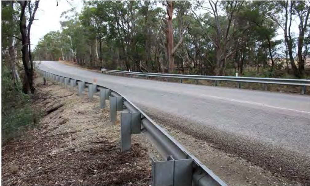
Road level looking south
