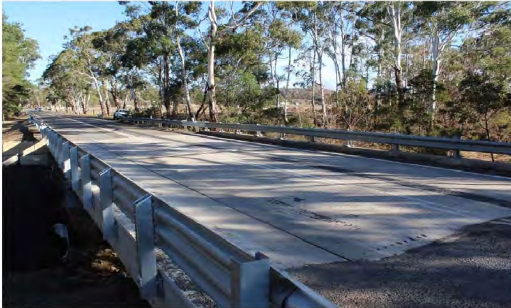
Bridge deck from north east
