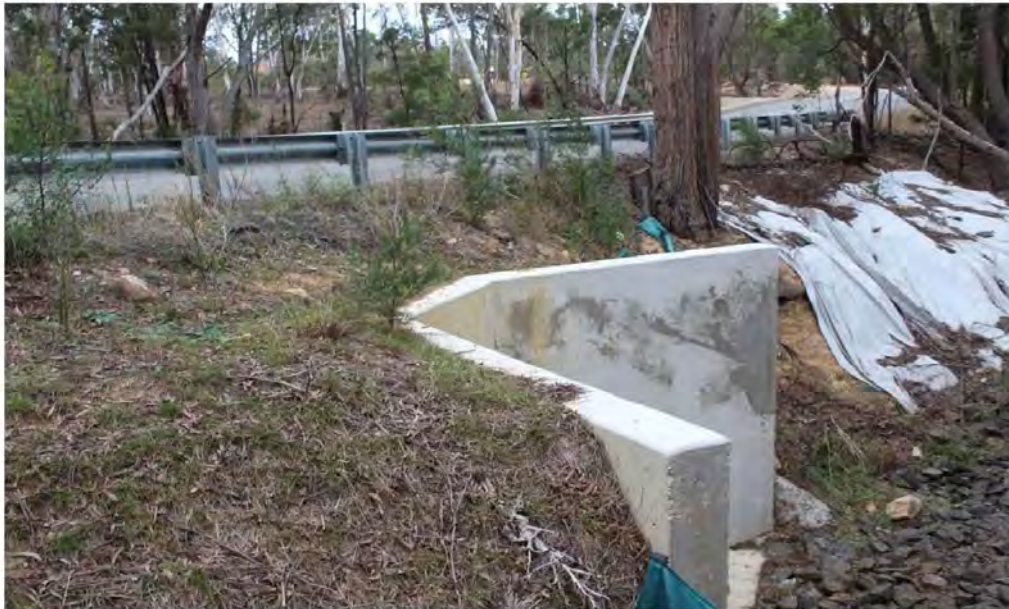
Pipe inlet (western side)
