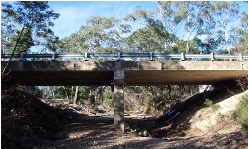
View of bridge from west
