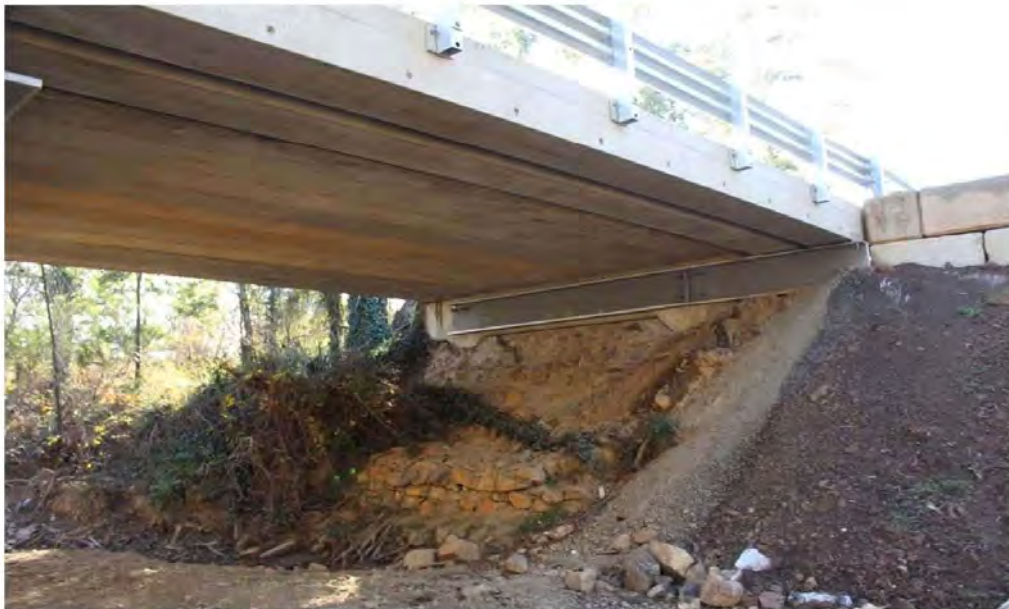
Abutment B and girders
