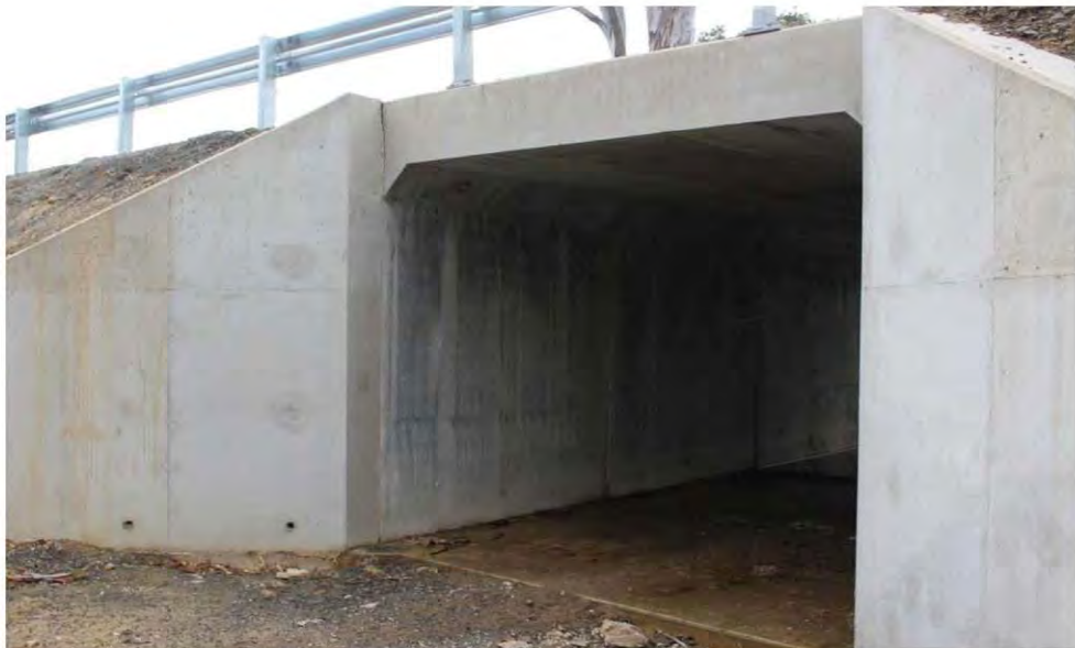
Side view of culvert
