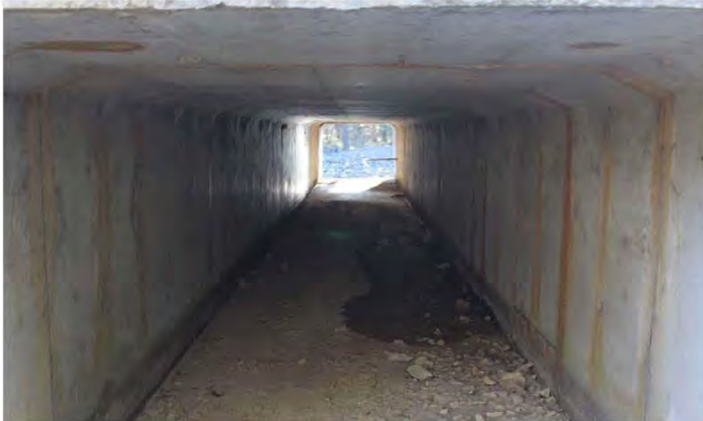
Inside culvert facing west
