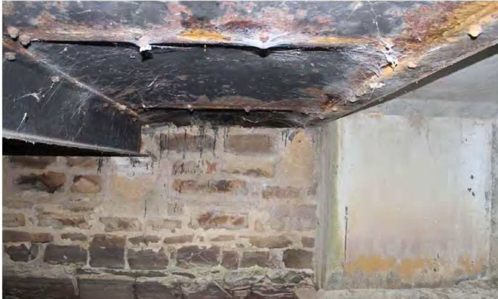
Beams 1 and 2, steel decking and eastern culvert
