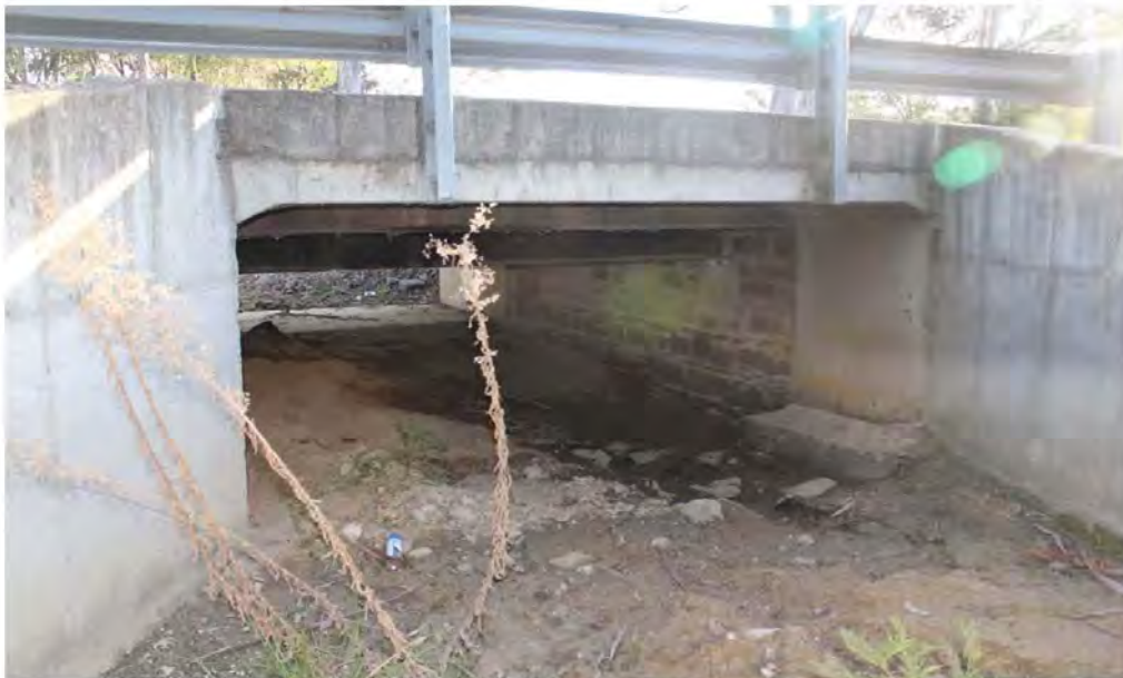
View from eastern side (including northern abutment)
