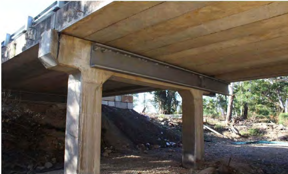
Pier from south west
