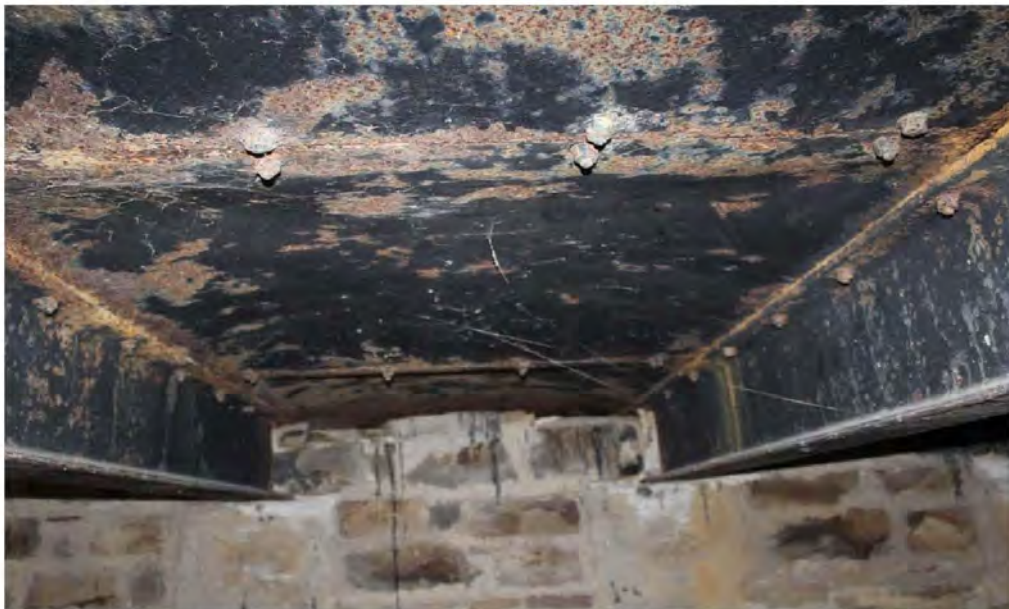
Beams 2 and 3 and steel decking
