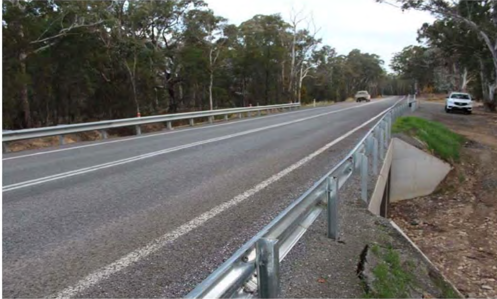
Culvert from road level (facing south)
