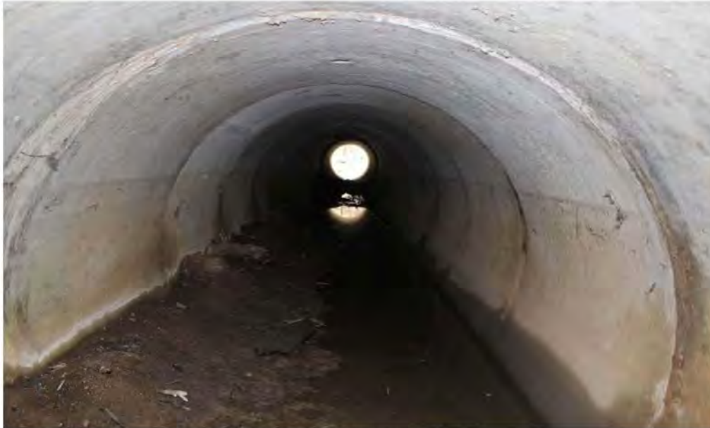
Inside culvert looking north
