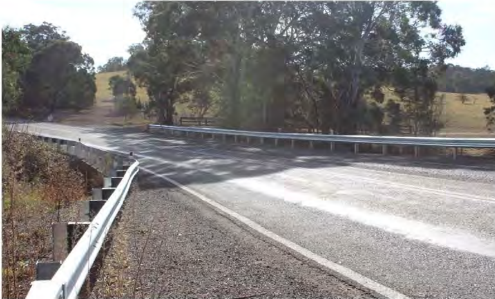
View of culvert at road level facing north
