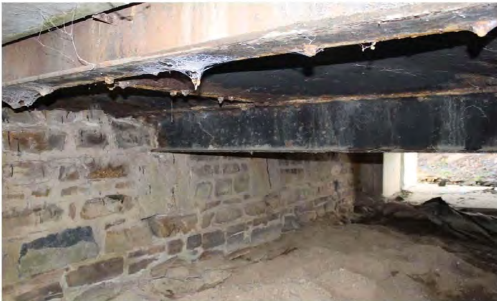
Southern abutment and beams 1 and 2
