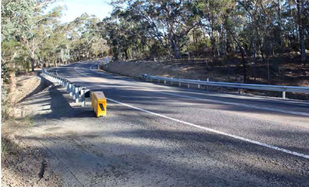
View of culvert from road level facing south
