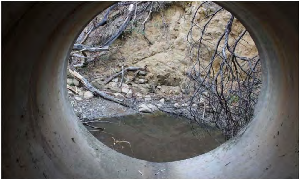
Pipe outlet (eastern side)
