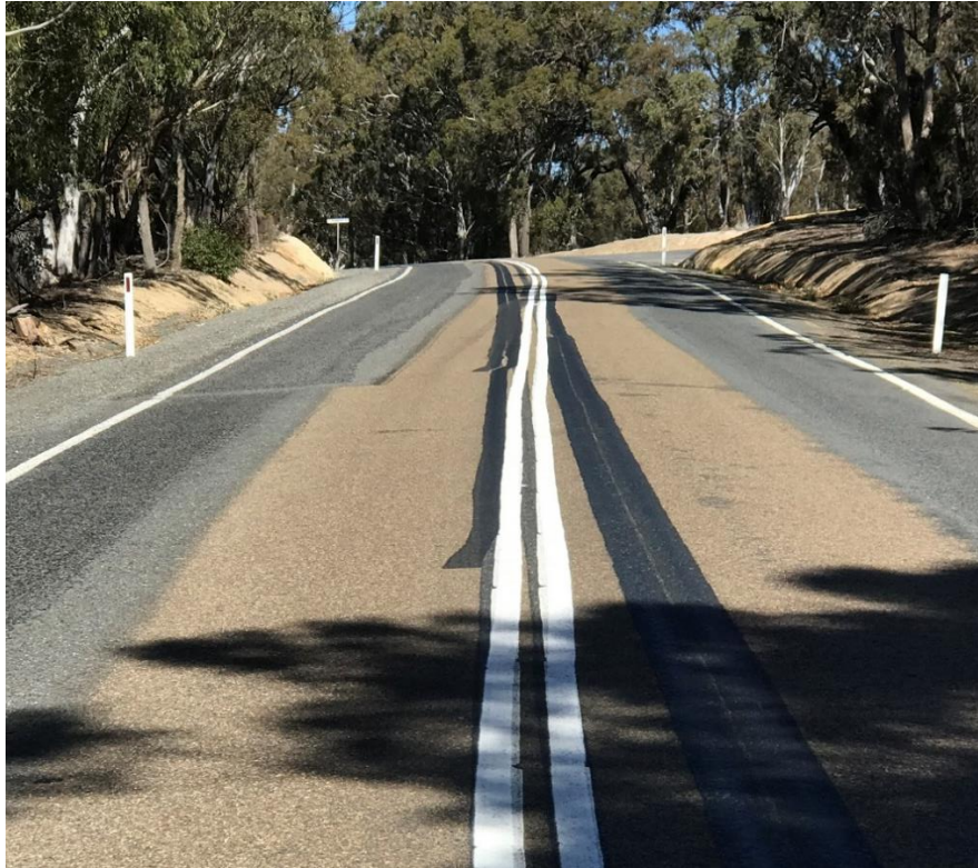
Blacking out of redundant centerline markings is not effective with sunlight reflection
