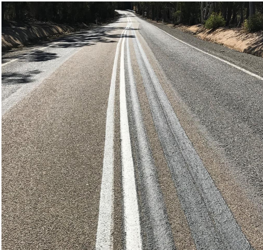
Blacking out of redundant centerline markings is not effective with sunlight reflection
