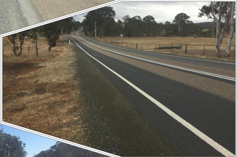
Plate 2: Pavement Widening of Jerrara Road 1 (Ref: Jerrara Road 1)
