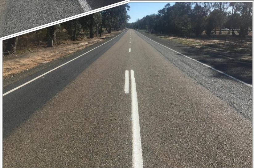
Plate 4: Pavement Widening of Jerrara Road 3 (Ref: Jerrara 2)
