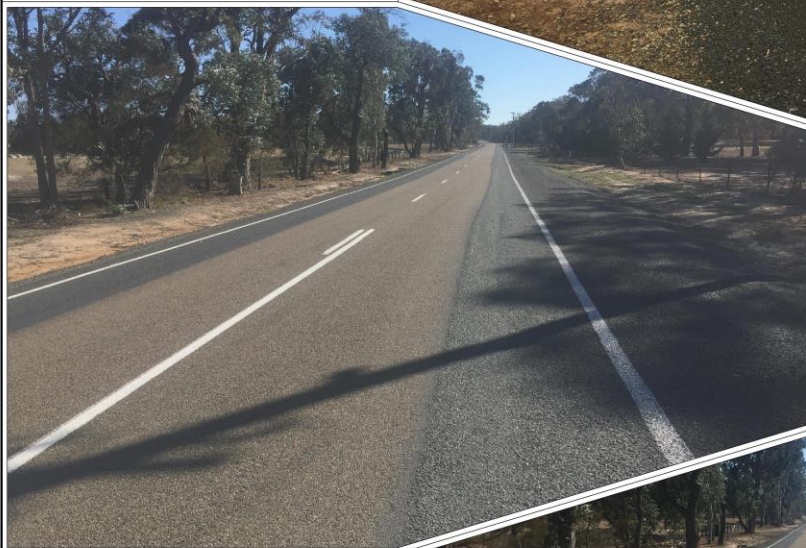
Plate 3: Pavement Widening of Jerrara Road 2 (Ref: Jerrara 1)
