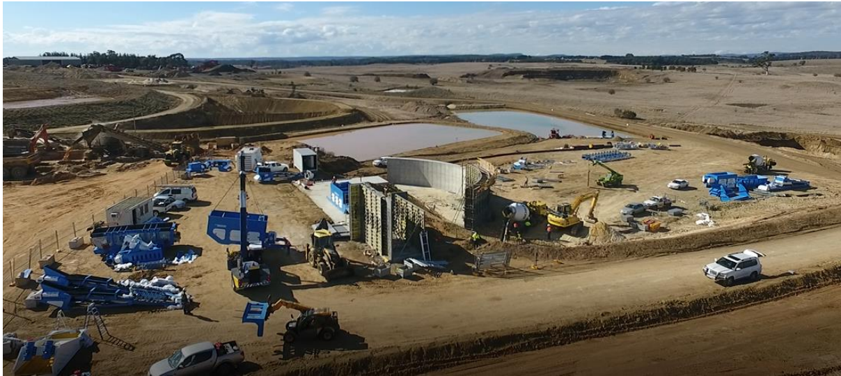
Figure 4 - Early stages of site preparation and plant installation
