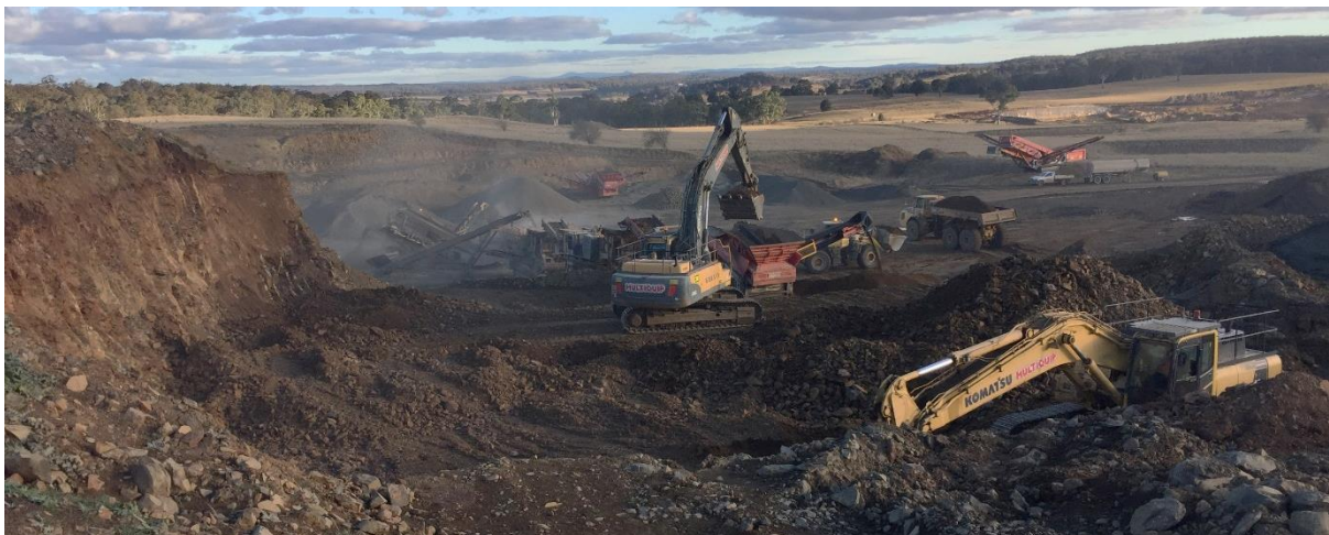
Figure 3 - Rock Extraction, crushing and screening
