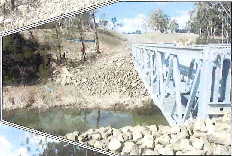
Plate 2: Bridge over Bungonia Creek, looking southeast (Ref: E625G_014)
