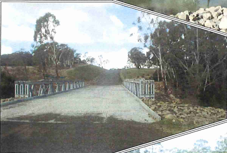
Plate 3: Bungonia By-pass road surface looking southeast (Ref: E625G_017)
