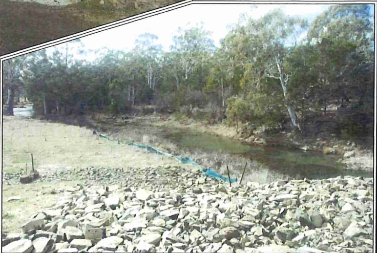
Plate 4: Sediment fencing adjacent to Bungonia Creek, looking northeast (Ref: E625G_013)
