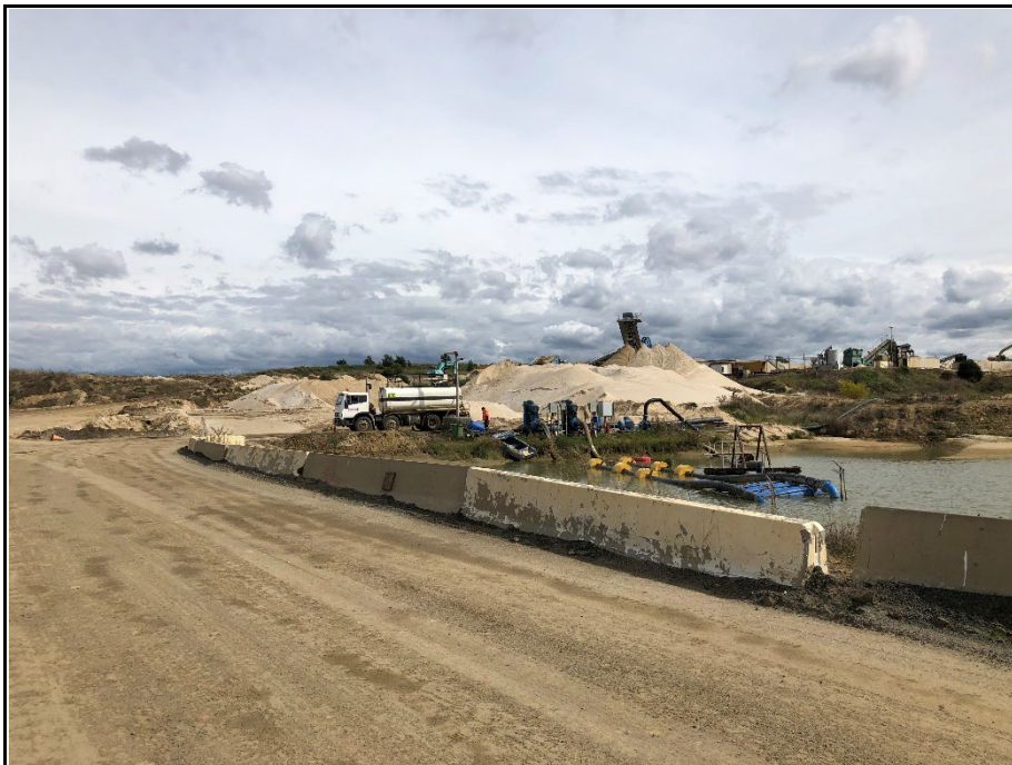
Photo 2: Sand processing and product storage, looking north west across Reuse Pond.
