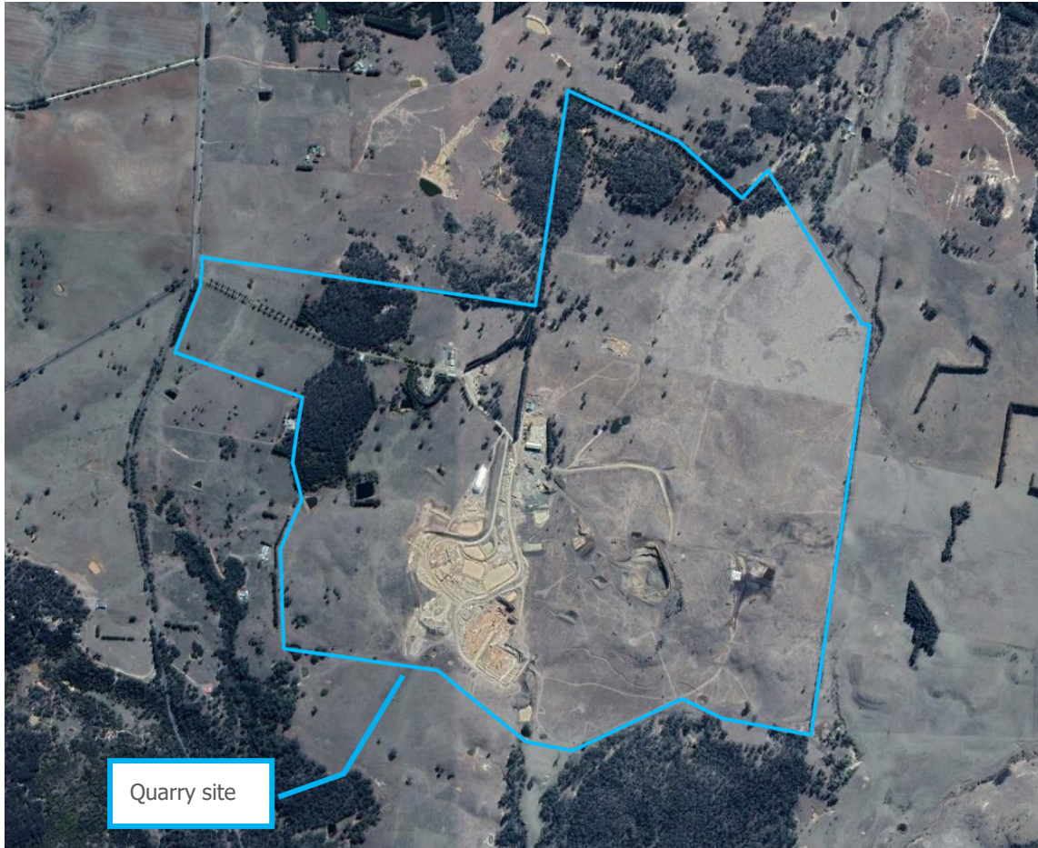
Figure 2-1 Ardmore Park Quarry Location
